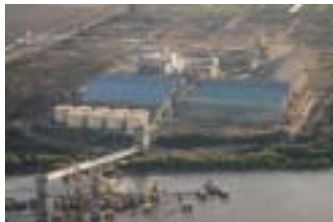
Cargill Soya Oil Processing Plant, Argentina
