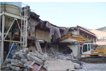
Demolition and decommissioning of the Barnices Valentine site in Barcelona
