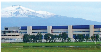
STMicroelectronics Plant, Italy
