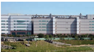
Chi Mei Optoelectronics Flat Panel Facility, Taiwan
