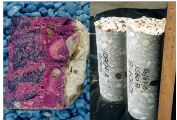
Advanced petrography testing on core samples is often used to determine the interface boundary between good and poor concrete
